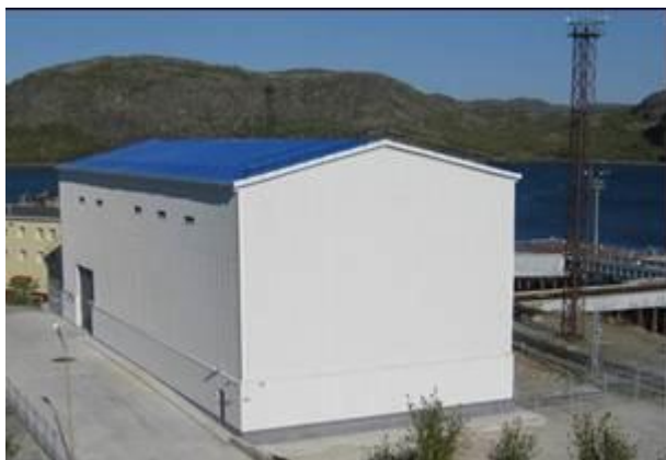
New Accumulation Pad for SNF Casks at Andreeva Bay
