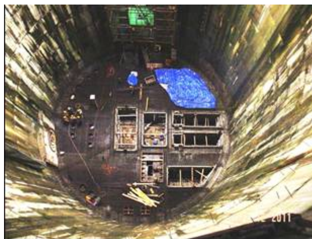
A 90m deep shaft built to house NDEP financed pumping station
