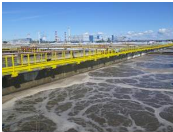
Modernization of the Northern Wastewater Treatment Plant is partly funded by NDEP
