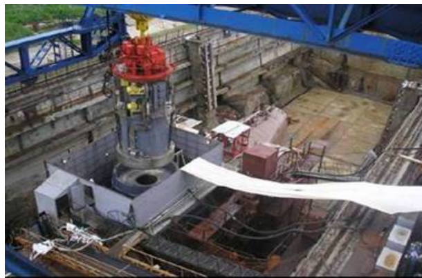
Alfa class reactor core unloading at Gremikha for further transportation to NIIAR
