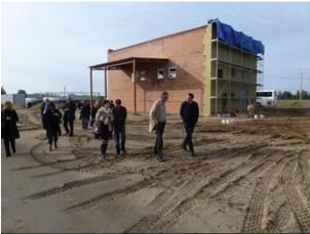
Sludge Dewatering Station approaching completion
