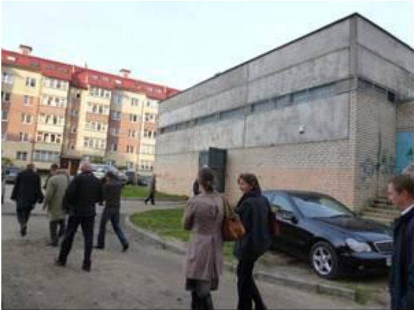
Outside a group heating substation financed by NDEP which provides hot water and heating to a housing estate in Kaliningrad
